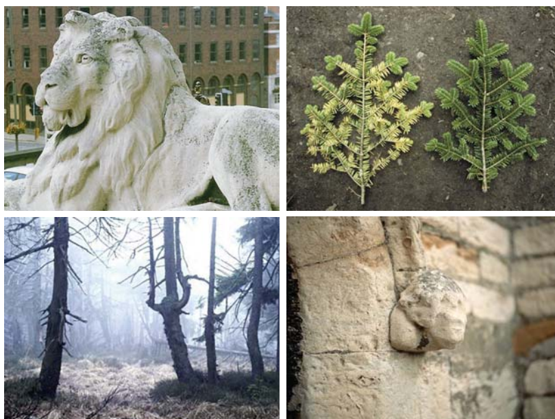
Damaged by acid rain
